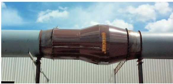
Q096, 8 foot diameter Quencher spark arrester
